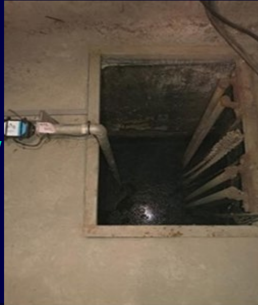
Sump Pit / Septic Tank Overflow (Dry Contact)
