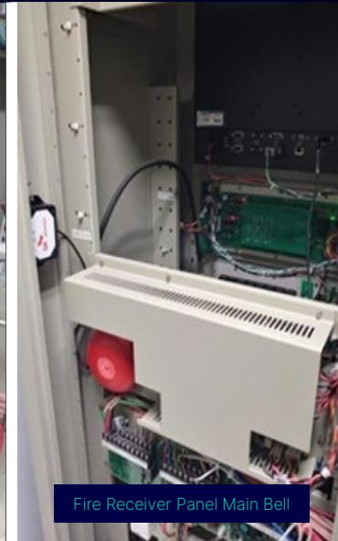
Fire Receiver Panel Main Bell Terminal
