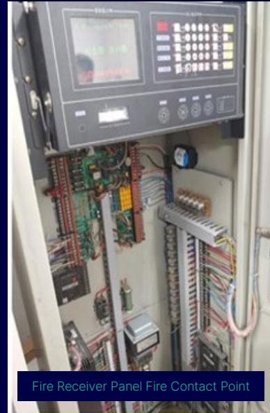
Fire Receiver Panel Main Bell Terminal
