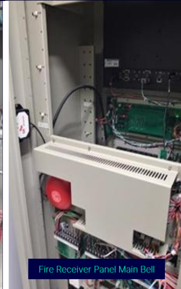
Fire Receiver Panel Main Bell Terminal
